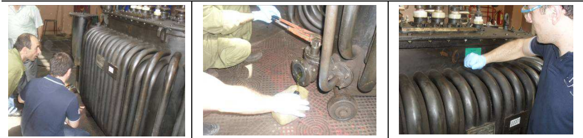
Facility: Yerevan-1 HPP “The International Energy Corporation”
